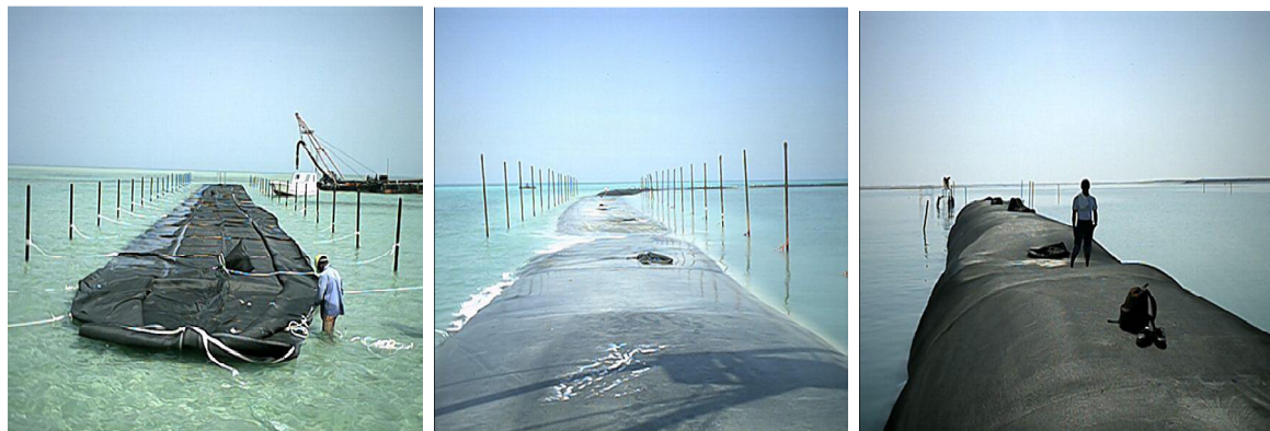
Figure 3-20 Example of Geotextile Breakwater Core Construction (Anwaj Is, Bahrain (Bergado, 2005))
