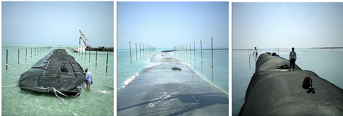
Figure 3-19 Example of Geotextile Breakwater Core Construction (Anwaj Is, Bahrain (Bergado, 2005))
