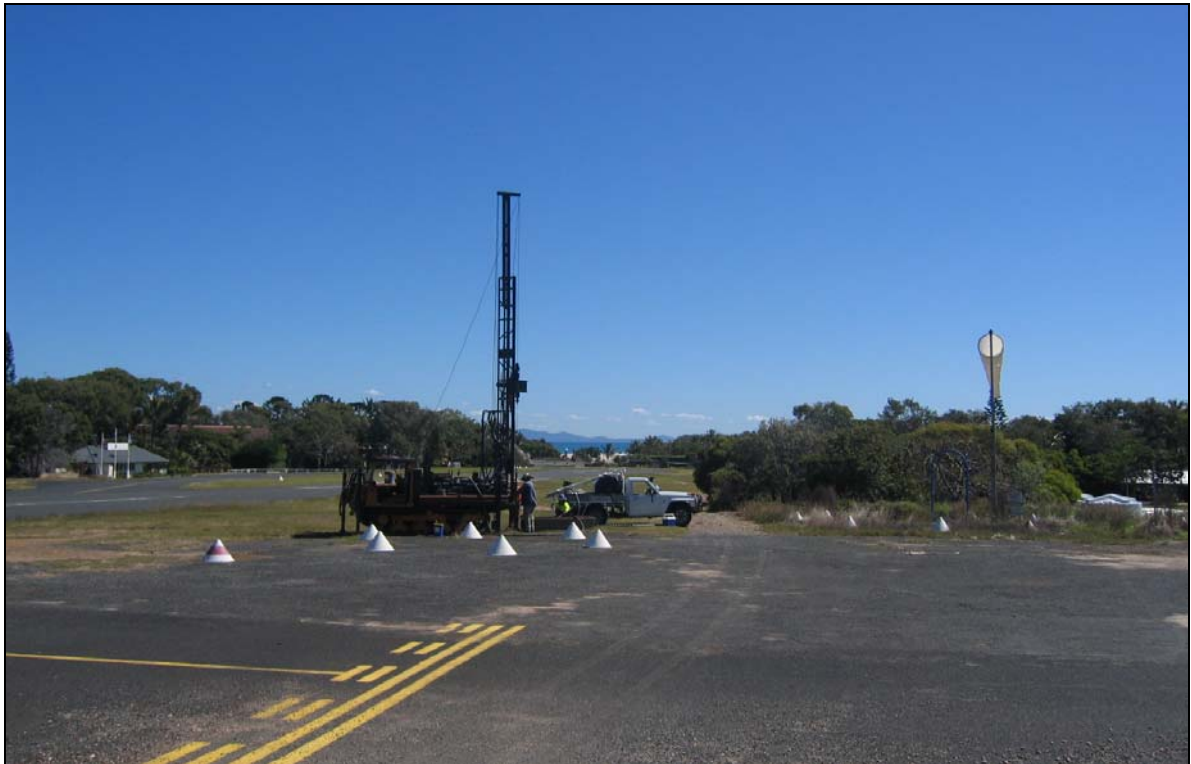
Photo 1: Drilling rig set up on Monitoring Bore 7 on the side of the airstrip.
