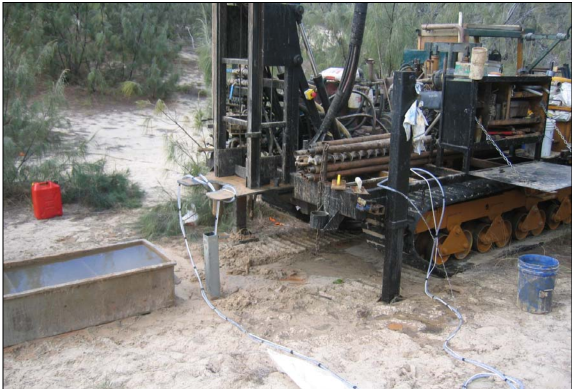
Photo 4: Pumping Monitoring Bore 5 to complete development prior to sampling.
