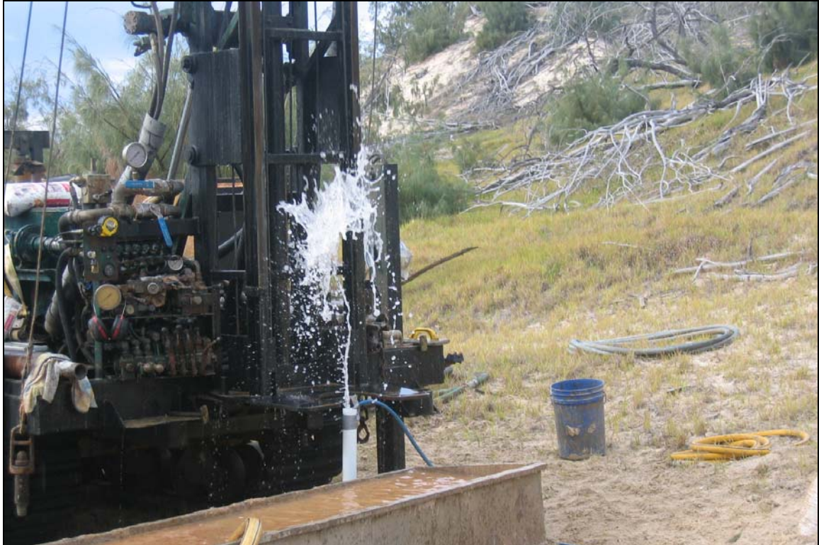
Photo 3: Airlift development of Monitoring Bore 4, Northeast Aquifer.
